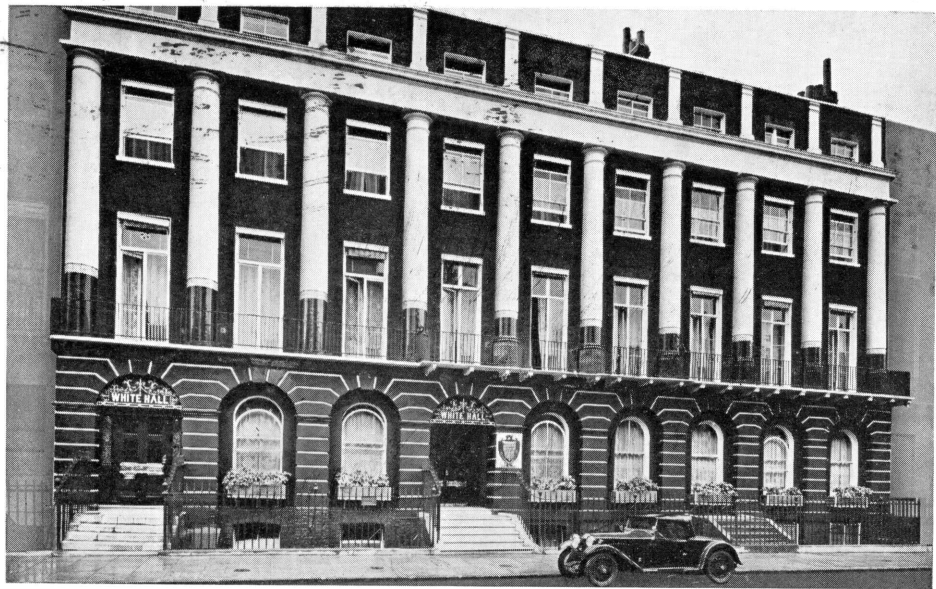
WHITE HALL, 70, 71, 72 GUILFORD STREET, W.C.1.
